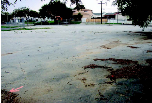
Stormwater Management Open Charter School, Los Angeles-Before
